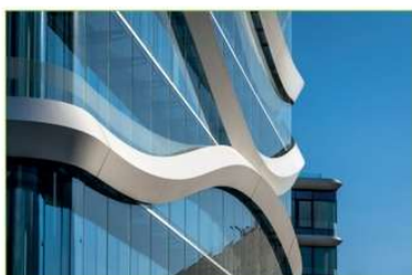
Fig. 2: Detailed view of the glazing and composite elements
