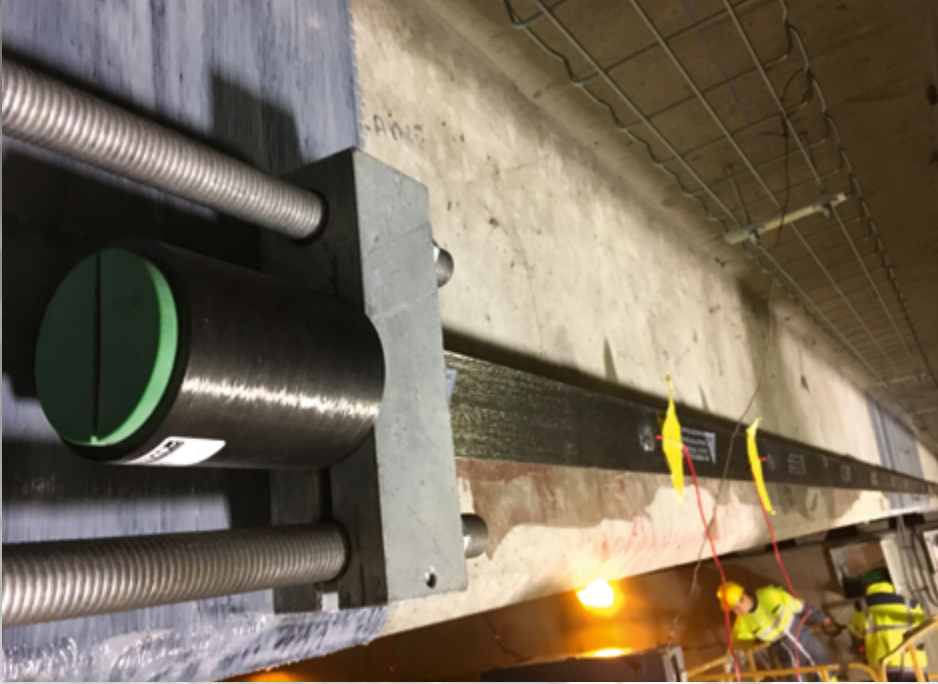
Pont de Pontcharra-sur-turdine, France Sika Carbostress® - SikaWrap®-230C
