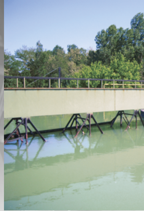
Papeterie Conda, France Sika CarboDur® S
